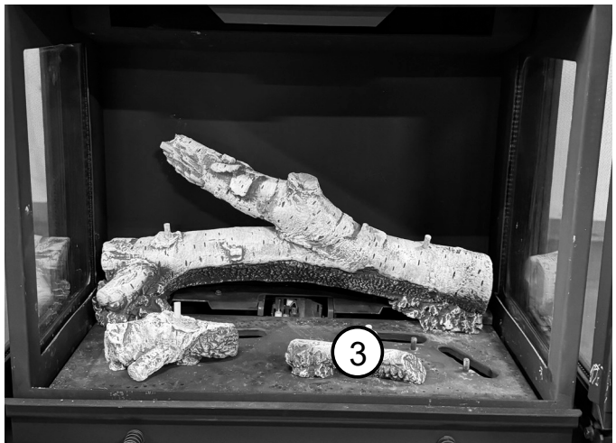
Figure 11.9. Place the #3 Middle Lower Log on the middle front pin.
