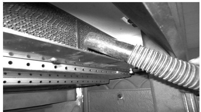
Fig. 18. Vacuum the combustor cells after brushing.
